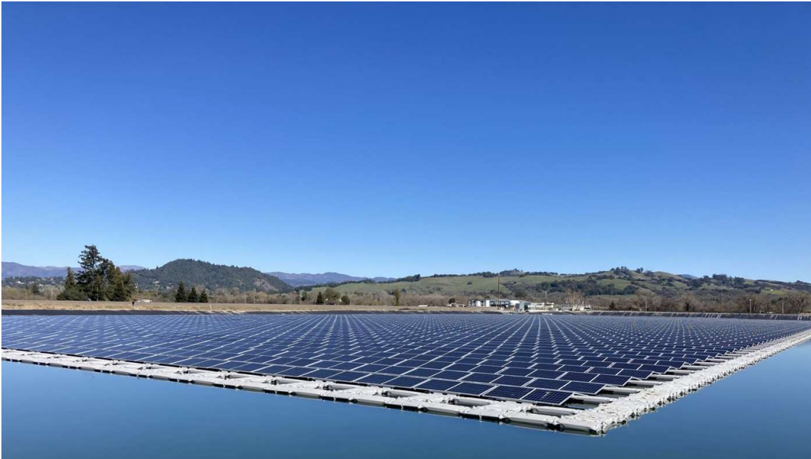
Picture7 floating solar power system "Aguasol" in Córdoba, Colombia 13
